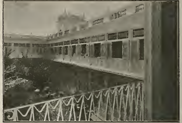
REAR VIEW OF THE BUILDING.
