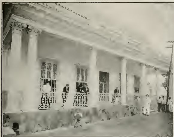
SIDE VIEW OF THE BUILDING.
